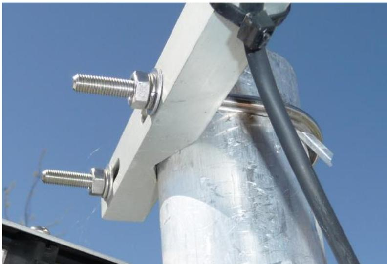
Figure 2-2: U-Bolt assembly and support arm attachment
